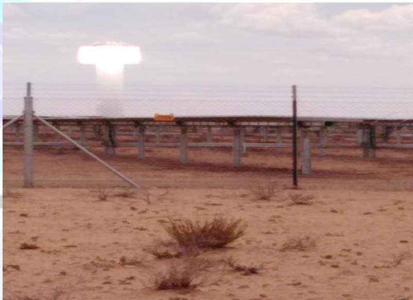
Capacitors & Transformers installations
